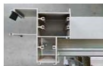
Check the connection with transom and mullion
