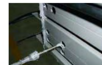
Nailing with sealant
